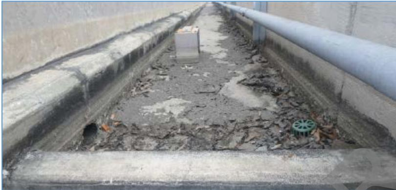
FIGURE 29: TYPICAL DECK DRAIN PLACEMENT
