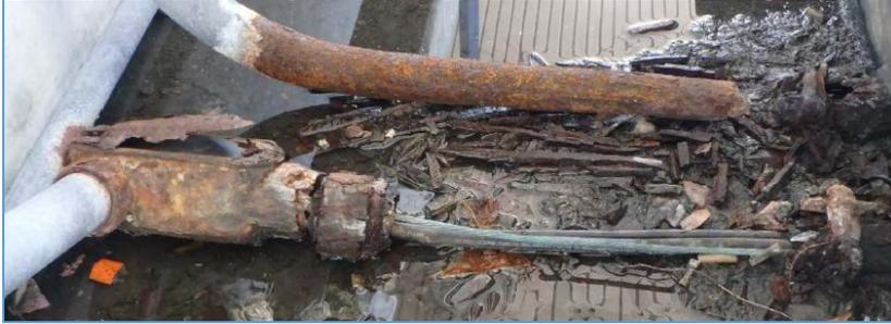
**FIGURE 39: CONDUIT CONDITION ALONG GUIDEWAY SECTION**
