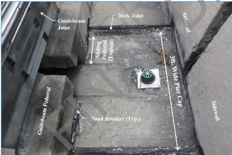
FIGURE 30: TYPICAL DECK DRAIN PLACEMENT
