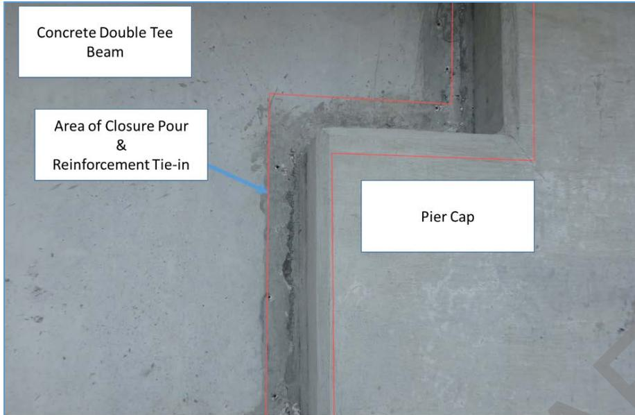
FIGURE 35: FIXED BEAM END DETAIL
