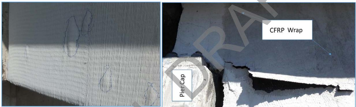
FIGURE 4: CFRP WRAP
