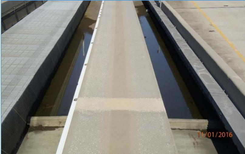
FIGURE 31: DRAINAGE BARRIERS (WEIRS)
