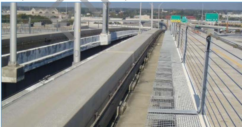
FIGURE 38: EXAMPLE OF POWER RAILS AND CONDUIT ATTACHED TO GUIDEBEAM, RIVER CROSSING
