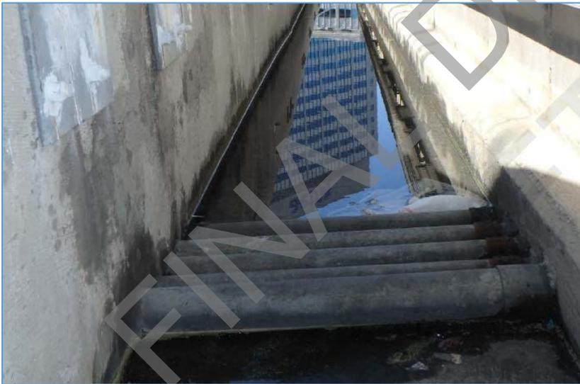
**FIGURE 41: EXAMPLE OF TRANSVERSE CONDUIT ALONG GUIDEWAY**
