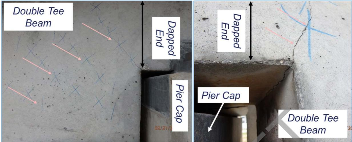
FIGURE 3: DAPPED BEAM END DETAILS
